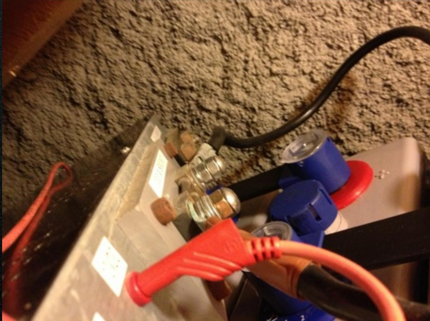
24 V, 390 Ah, 9.3 KWh, Pb-H<sub>2</sub>SO<sub>4</sub>
